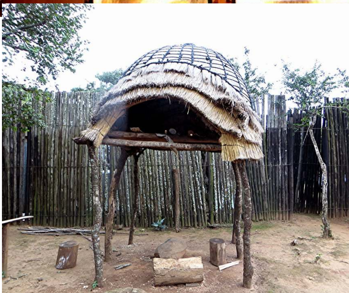
Shown on the left is a full sized food storage hut supported on four tree limbs to keep the food out of reach of stray animals.
